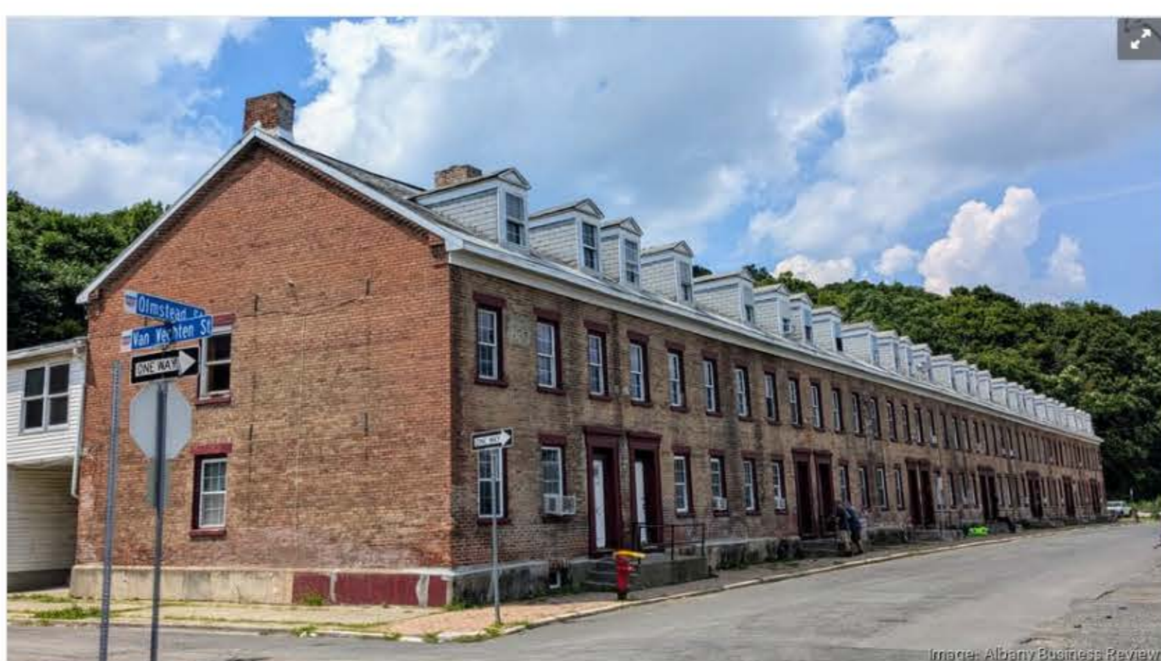
The row of apartments is a short walk from Remsen Street in downtown Cohoes. DONNA ABBOTT-VLAHOS / ABR
